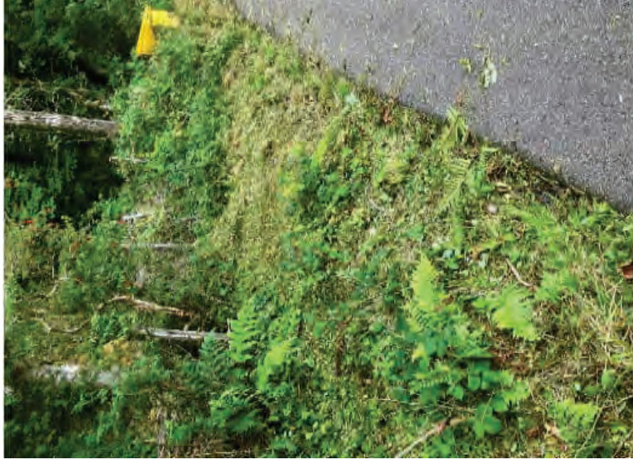
View down the private access road in the direction of Polvinister Road
